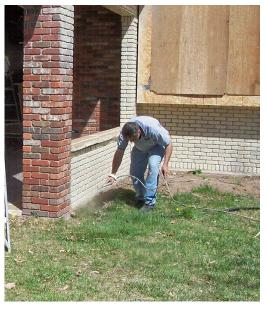
use on masonry. They have perm ratings of 9 or 10. A high perm factor indicates a paint with a high capacity to transmit water vapor.
