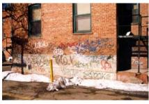
All types of cleaning are hard on masonry walls. Cleaning should only be attempted if the layer of dirt is actually harming the wall. Acid rain trapped at the face of the wall by encrusted dirt can eat away at the face of the brick. If cleaning is necessary, do several tests to determine which cleaning procedure and solution will be most effective. Choose the gentlest method which
