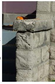
The patch must be softer than the surrounding stone to ensure that the repair does not deteriorate the wall further. If reinforcement is used, it should be non-corrosive. Stainless steel reinforcement is best.
